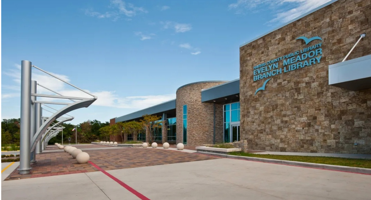
ENGLISH ARCHITECTS' EVELYN MEADOR BRANCH LIBRARY, HOUSTON'S FIRST LEED GOLD CERTIFIED LIBRARY
